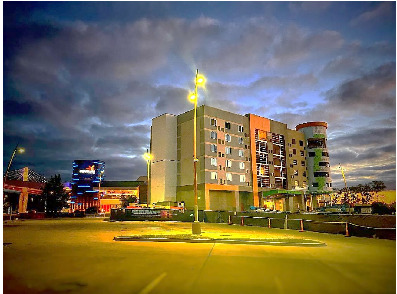
Cape Girardeau Hotel Construction Progress
